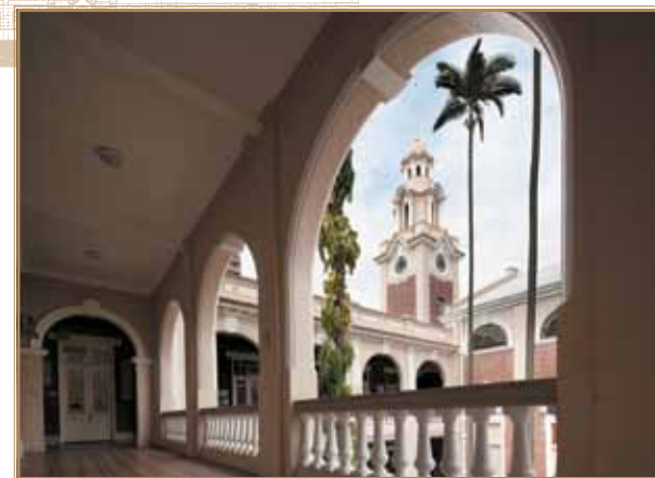
MAIN BUILDING Opened in 1912 Declared a monument in 1984
