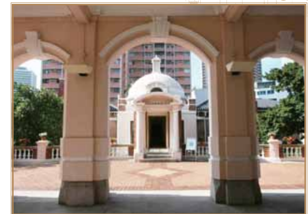
HUNG HING YING BUILDING Opened in 1919 Declared a monument in 1995
